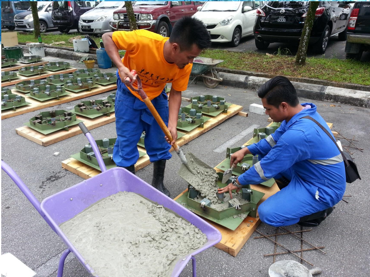
First mass casting in February 2015
