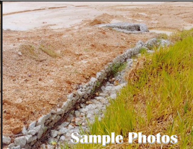
Earth drains laid with gravel
