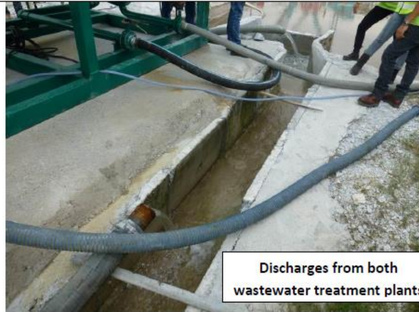
Both wastewater treatment plants with capacity of 80m 3 /hour at Pasar Rakyat Station Site
