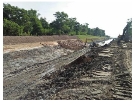
Excavation at site to remove existing soil
