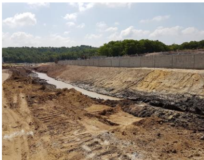
Existing slope at site
