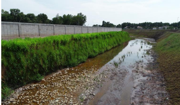
Reinforced soil slope with green surface
