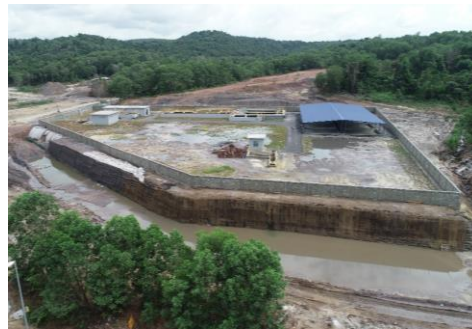
Overview of reinforced soil slope
