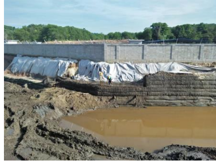
Steel mesh is used to form a 60° slope angle
