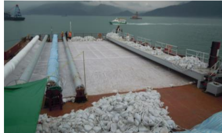
Placement of conventional geotextile for bedding
