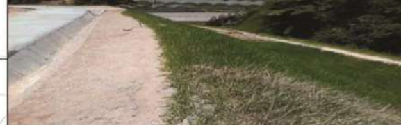
Road 12, roadside drain and hydroseeded slope at plot 2
