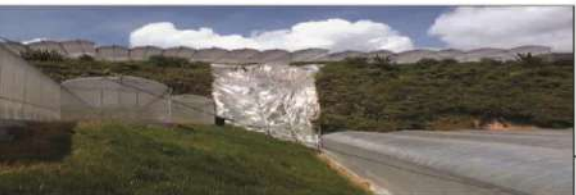
Part of slope at Plot 38 is covered with plastic sheet
