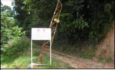
Northwestern entrance to the Project Site
