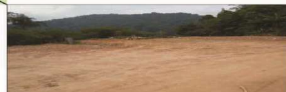
Land preparation at Plot 36
