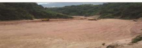
Land preparation at Plot 32
