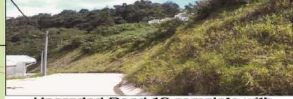
Upgraded Road 19 complete with roadside drain and streetlighting
