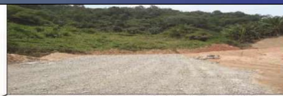
Aggregates are laid at Road 12
