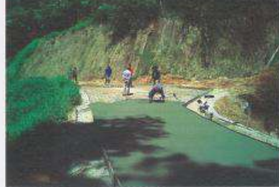
4.) CONCRETED ACCESS ROAD
