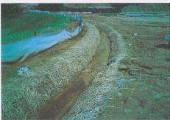
1.) TEMPORARY EARTH DRAIN
