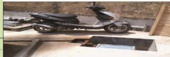
Oil Interceptor at genset storage area
