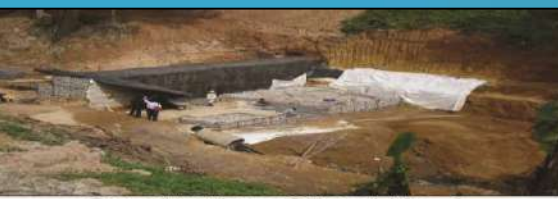
Construction of Pond No. 4
