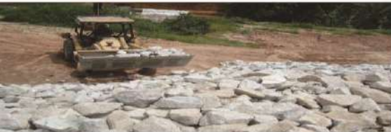
Stone aggregates for Dam of Pond No. 4
