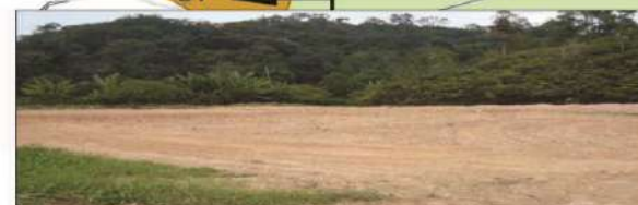
Land preparation at Plot 37
