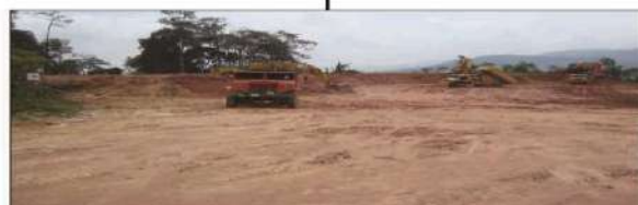
Land grading works at Plot 38
