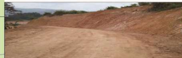
On-going upgrading works of Road 18
